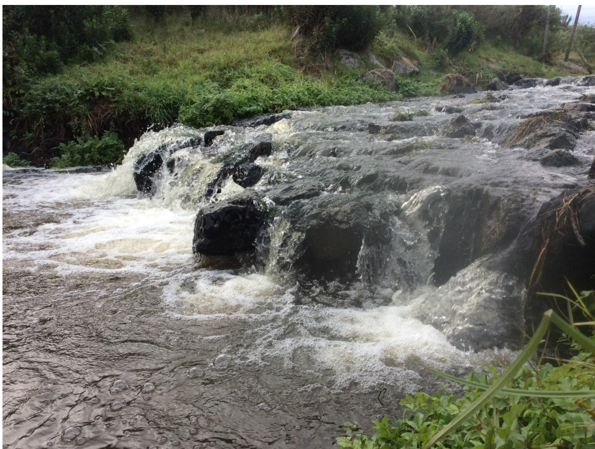
Figure 3: Previous fish pass fix on the Vector gasline. The constructed fish pass has created another perch due to sand substrate downstream. The perch disappears on during the high stage of the tidal cycle.
