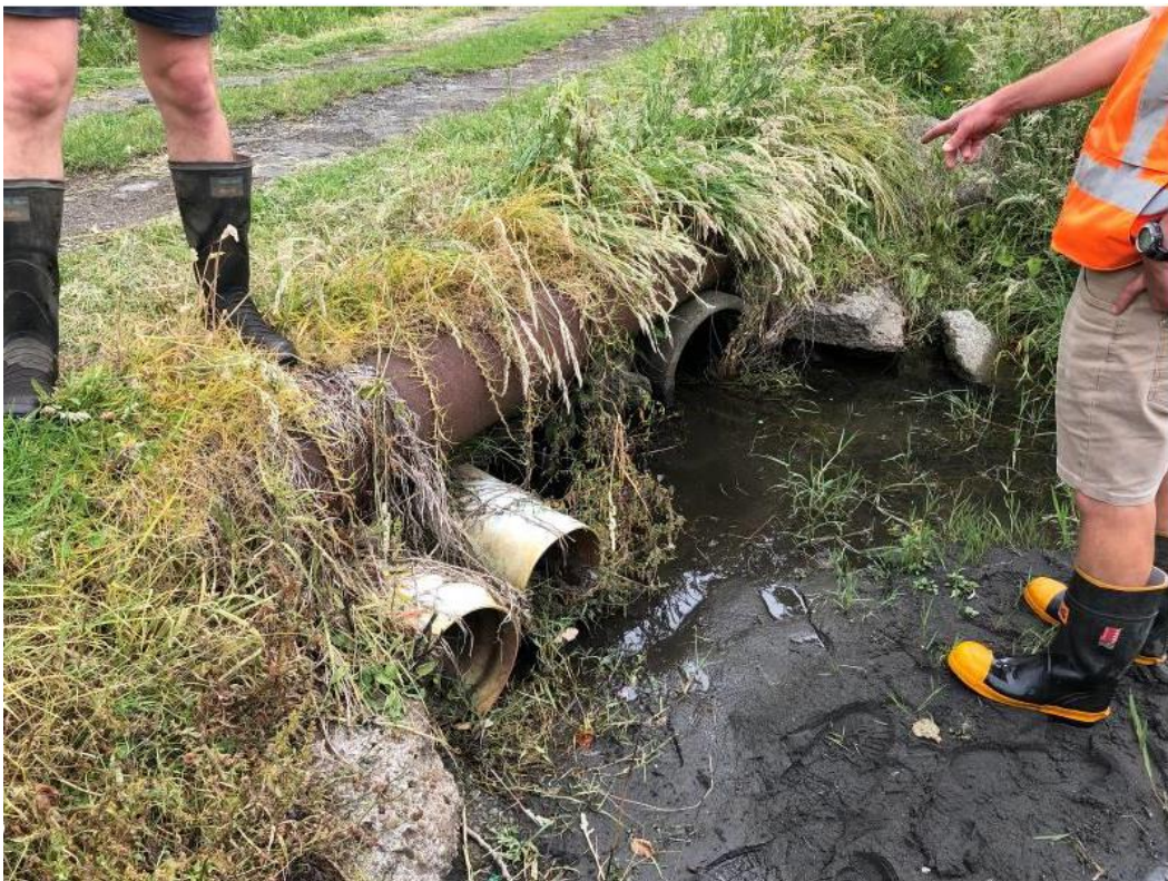
Figure 2: Access way and culverts – photo taken on the same day as Figure 1 (note sediment deposition in front of the culverts creating a mound for water flow).
